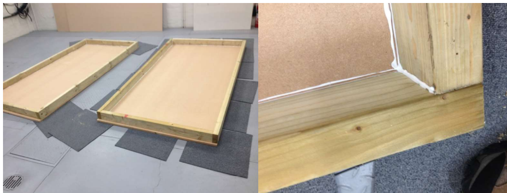
Figure 3: The absorbers under construction
