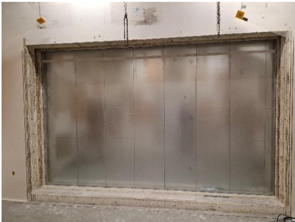
Figure 2: Installed wall assembly.
